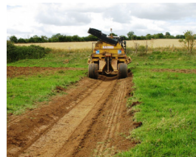
Foot drain creation with rotary ditcher
