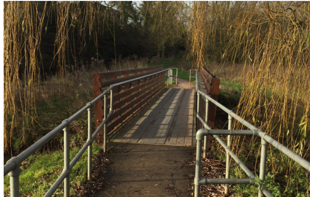
Pedestrian entrance to site with bespoke footbridge
