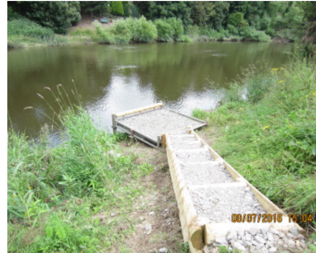
Fishing platform installed with timber steps
