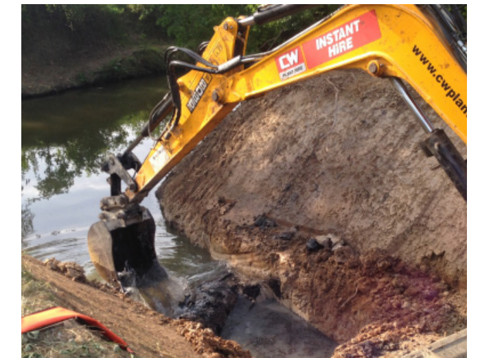
Excavating the backwater
