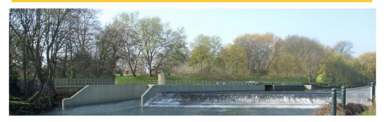
View of the proposed hydro scheme from Sydney Avenue. The turbine is situated below the small tower. The new fish pass will be between the weir and the hydro.
