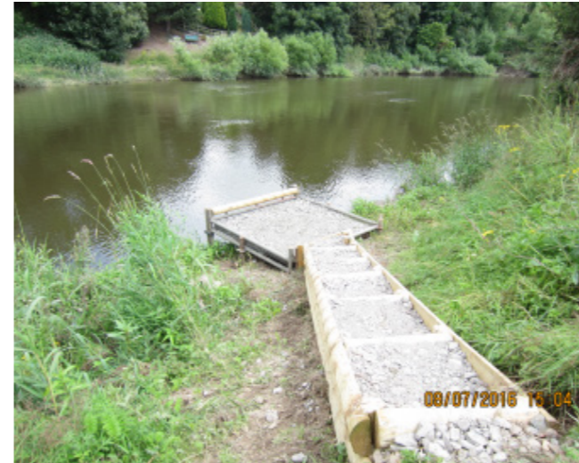
Fishing platform installed with timber steps
