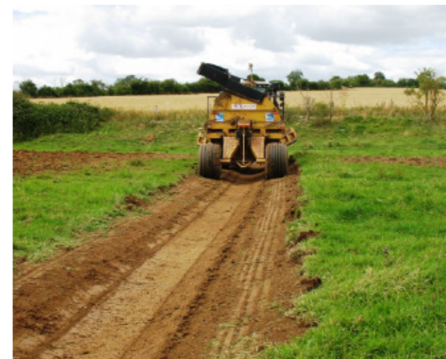
Foot drain creation with rotary ditcher
