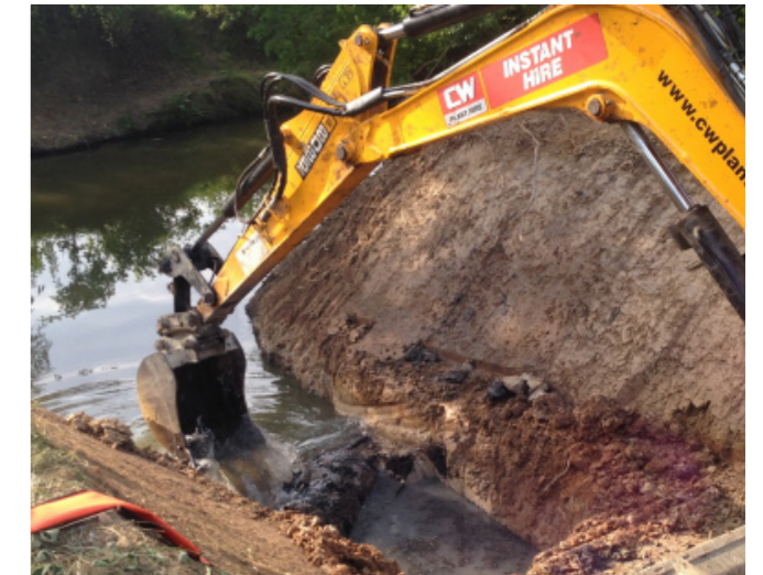
Excavating the backwater
