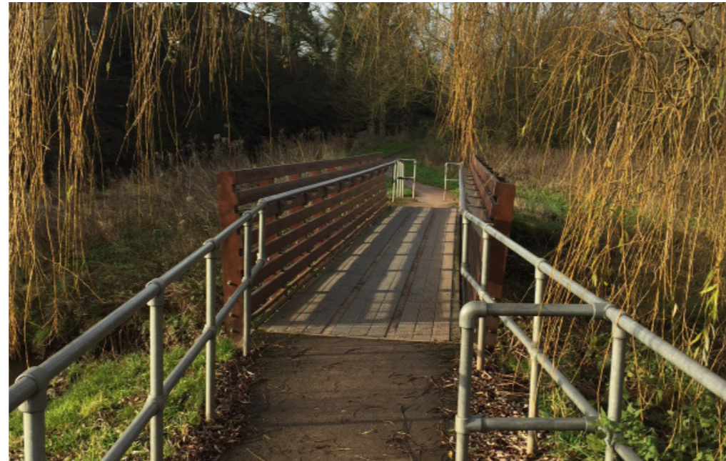
Pedestrian entrance to site with bespoke footbridge
