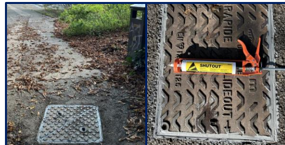
Shut Out Manhole Sealing
