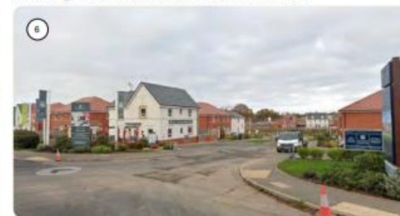
Neighbouring DWH/Barratt development under construction
