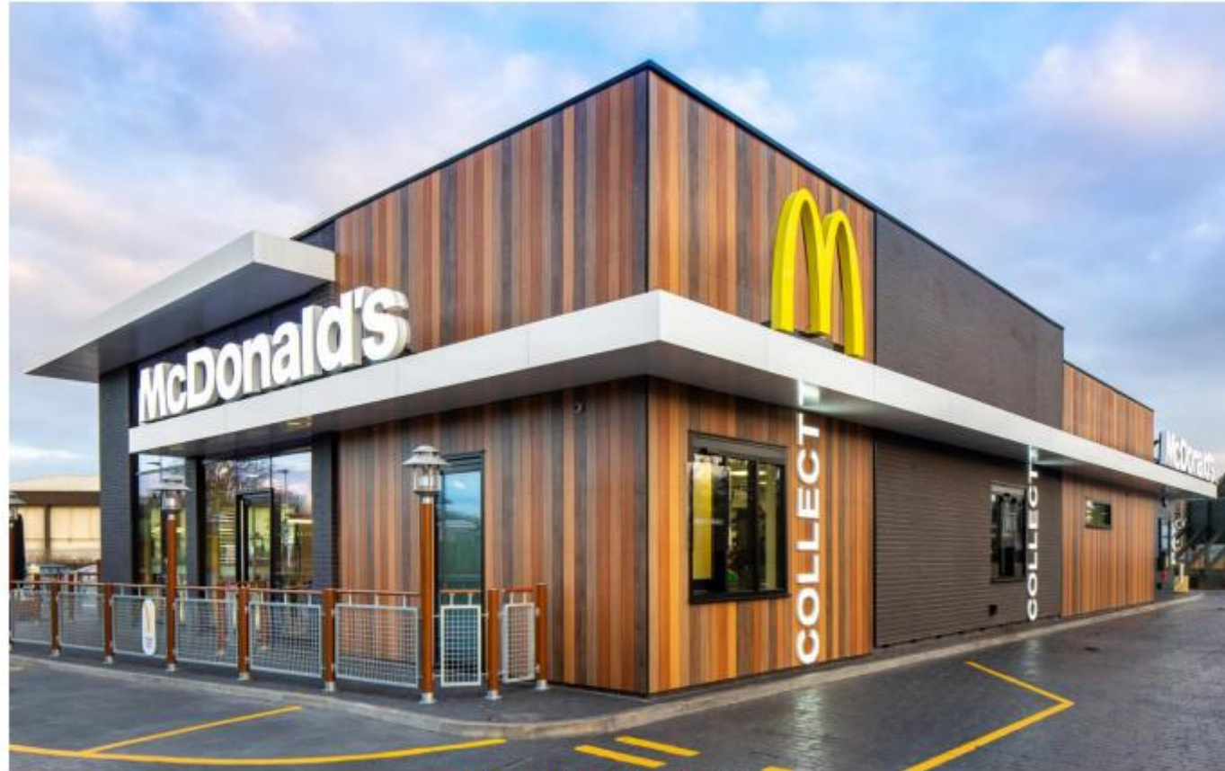
Example of the building
