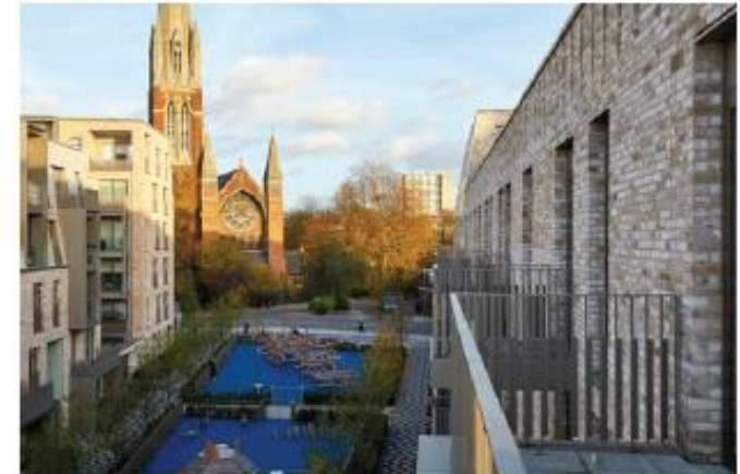
Figure 73 Balconies can project up to 2m and should be fully integrated in the design of the building.
